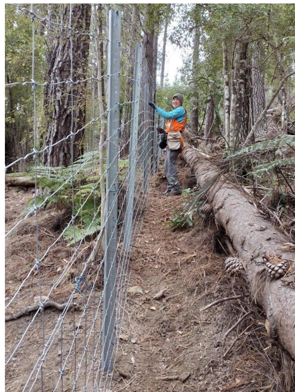
A 1.9m high ungulate exclusion netting fence constructed within the canopy control trials to compare browsing pressure on planted and naturally regenerating understorey, Maitai Forest, Nelson.
